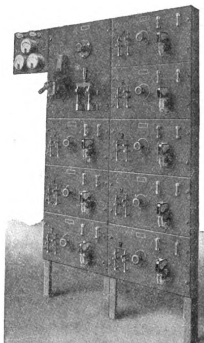
TYPICAL BATTERY-CHARGING SWITCHBOARD
